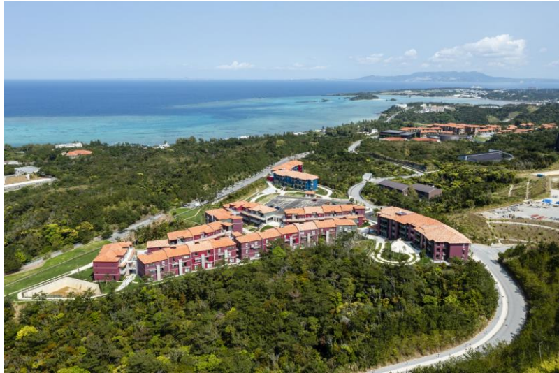
Aerial view of 'The Gardens' housing
