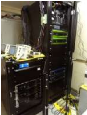
Left: Li-ion charger Right: DC power converter (Rectifier & DC-PCS)
