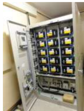
Flame-retardant Li-ion Battery (23 kWh)
