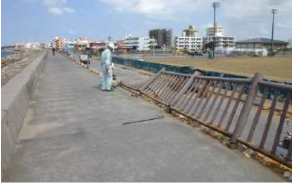
Bank damaged by high wave (Mizugama, Kadena town)
