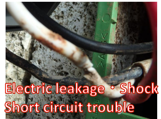
Damaged wires
