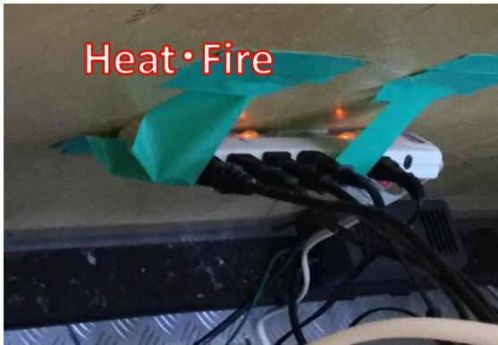
Overloaded power strip
