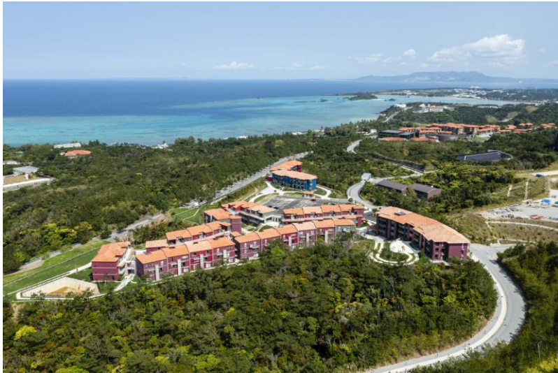
Aerial view of 'The Gardens' housing
